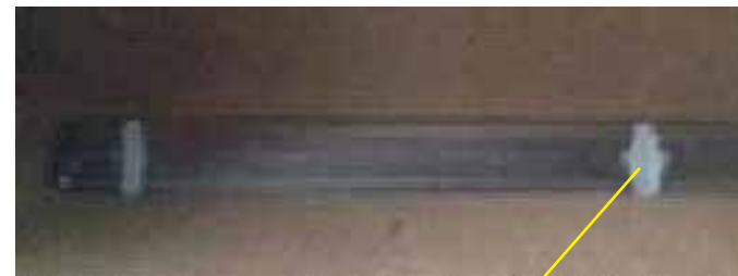
Fuel Oil Level Mark
