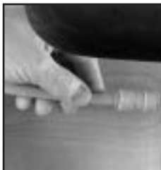
Completely insert 3/8" polyethylene tubing from outlet side of filter head into 3/8" to 1/4 quick-connect union fitting.
