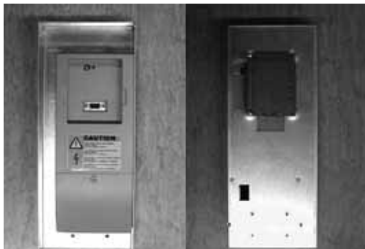
Figure 4-14: Control Unit Installed into the Mounting Box; Left: Front; Right: Back
