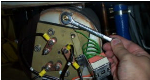
Removing the imperial brass fitting (Tempstar).
