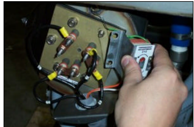
Removing the thermostat bracket.
