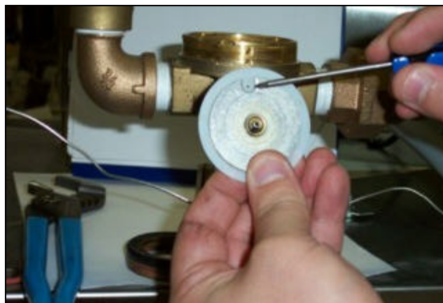
Pointing out the extension hole
