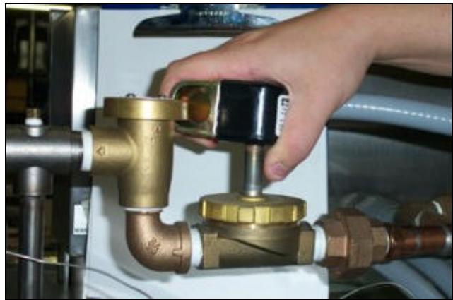
Removing the coil
