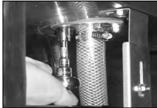
Removing the rinse drain weldment
