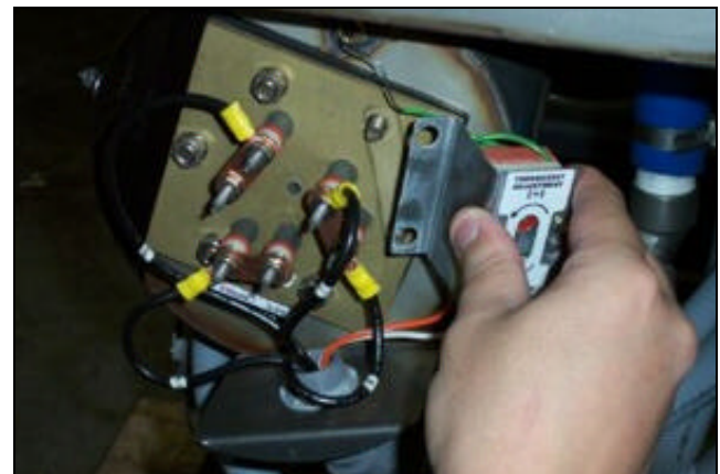
Removing the thermostat bracket.
