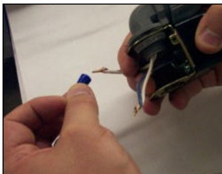
Removing the wire nuts
