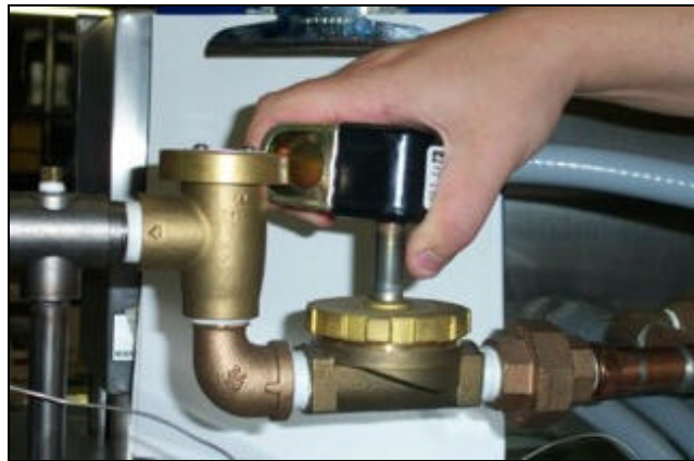
Removing the coil
