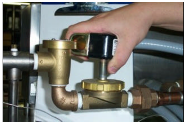
Removing the coil
