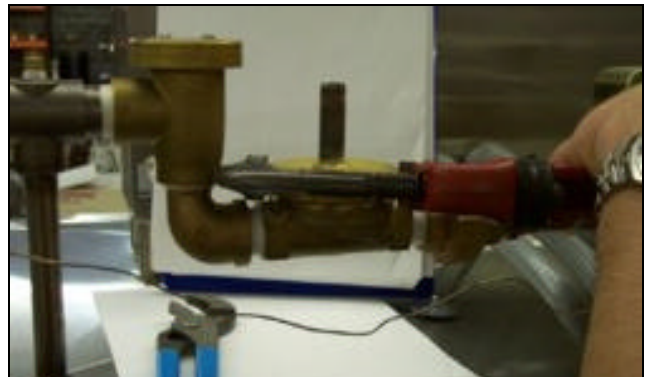
Loosening the valve bonnet
