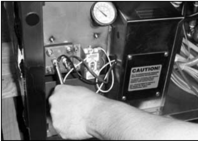
Removing the heater nuts.
