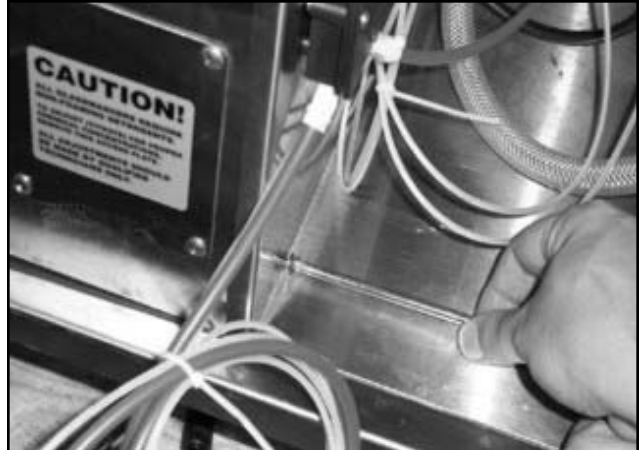
Removing the screws for the electrical box cover.
