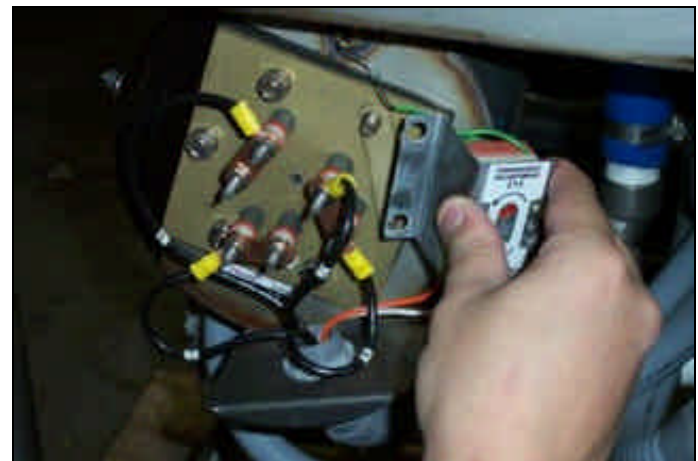
Removing the thermostat bracket.
