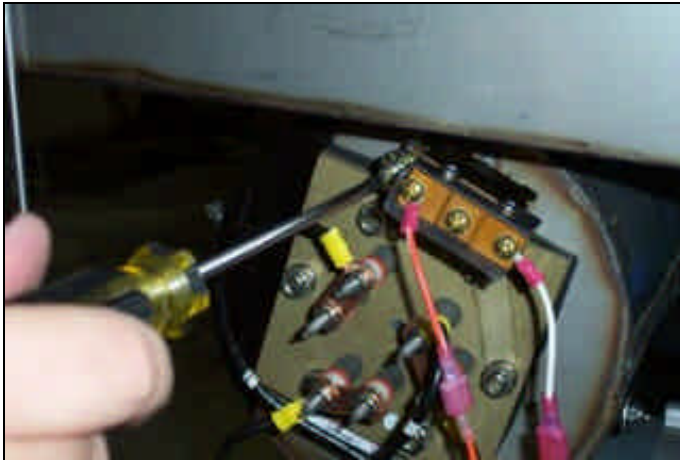
Calibrating the new thermostat.
