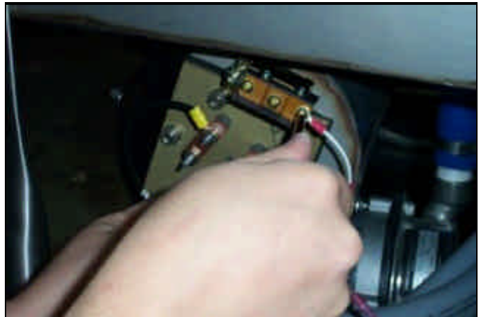
Securing jumpers to the thermostat.
