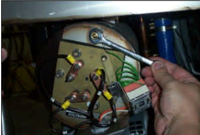
Removing the imperial brass fitting.
