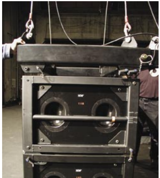
Figure 14. The MTG-3D Top Grid positioned over the first M3D block
