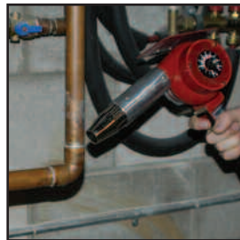
Solder Copper Pipe
