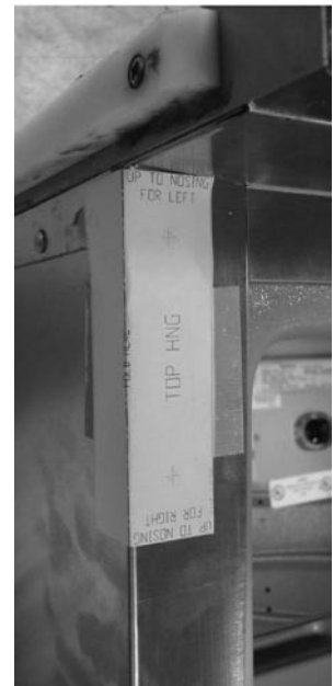
Top hinge template up to unit nosing
