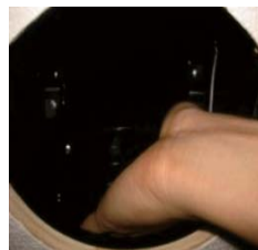
Move the casing section to the hole position
