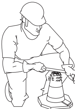
Figure 60-D. Slump Test (Removing Excess Concrete)
