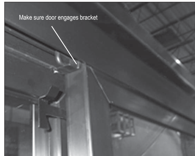
Figure 5. Removing/Installing Sliding Door
