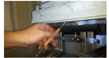
Picture 2 Use a small diameter rod (1/8" max.), or a Philips screwdriver to reach through the access hole and press the reset button.
