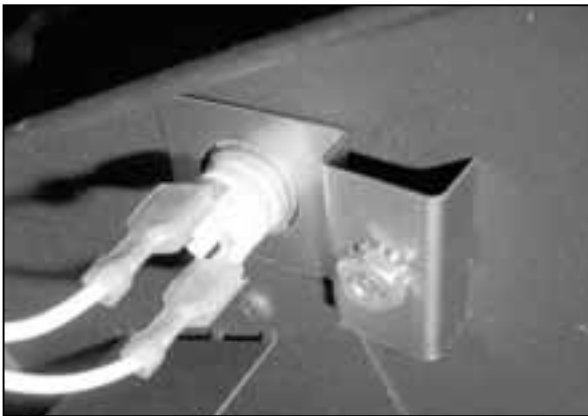
Figure 8.13 With the cast iron front of the appliance removed, remove the decorative cover located under the appliance. To remove the cover, remove the two screws on the front of the appliance that hold the cover in place. Pull the cover forward, down and out.
