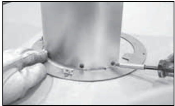
Figure 5.33 Attach the heat shield to the trim ring with the four screws provided. Screws go through the heat shield and into the brackets on the trim ring.
