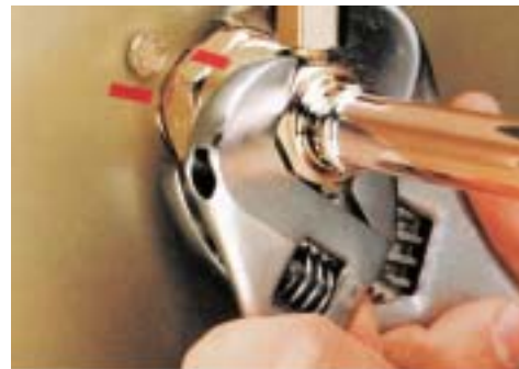
Rotate Swivel Nut \frac{1}{4} Turn More
