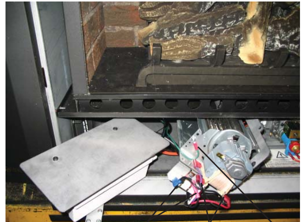
Resistor Con-nectors Fan Connectors Fan Ground Cable
