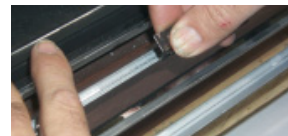
Push hold-down clip onto inside louver and press tab until it is at 90° to louver.
