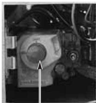
GAS COMBINATION CONTROL VALVE
