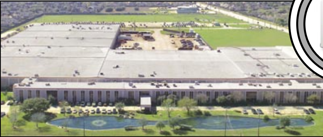
North America Headquarters and Manufacturing Facilities (Houston, TX)
