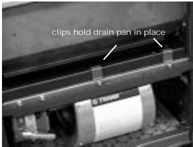
Figure M-MP-3. To remove the main drain pan on vertical fan-coil units, disconnect the clips holding the pan to the fanboard.
