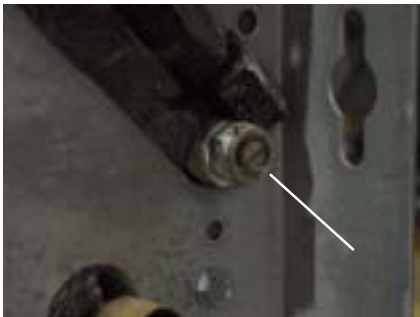
Figure I-MR-5. Manual coil air vent with set screw
