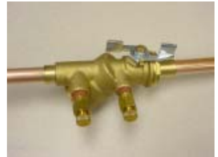
Figure I-MR-9. Automatic circuit setter valve
