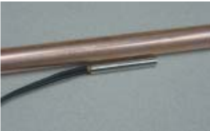
Figure I-MR-4. Close-up view of the changeover sensor
