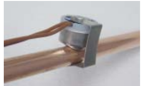
Figure I-MR-7. Electric heat lock out switch installed
