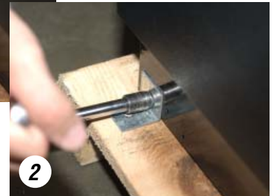
2 Removing bracket from cabinet.
