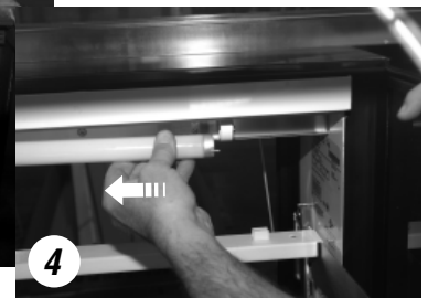
4 Remove bulb by gently pushing bulb into spring loaded lampholder.
