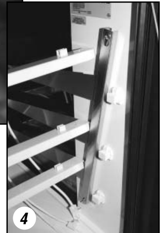
4 Install rear brackets.
