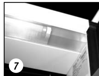
7 Interior top light assembly properly installed.
