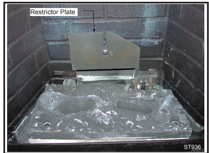
Fig. 9 SDDVR/SDDVRC restrictor plate.
