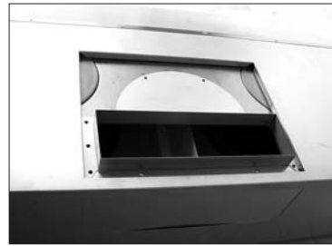
D. Overlap the rectangular starting collar on the top of transition plate.
