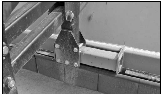
Figure 40. Strut Uprights Installed
