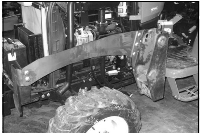
Figure 6. Left Side Rail Installed
