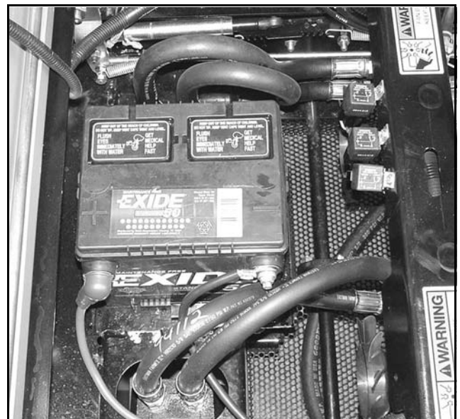
Figure 9. Battery Located under Seat
