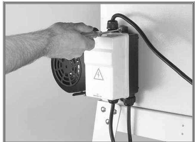
Figure 38. Installing magnetic switch.
