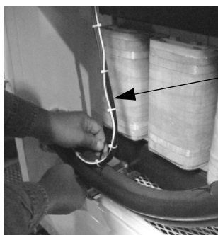
Figure 3-13 Tie-wraps on the AC Sense Harness
