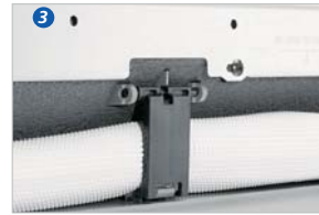
Additional wide cover to hold tubing assembly
