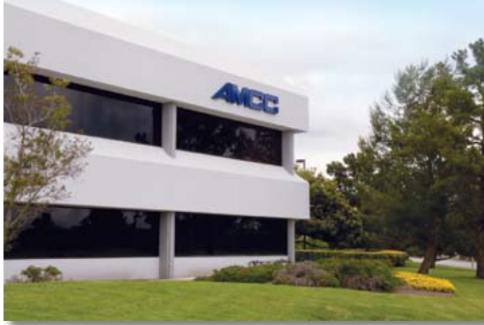
AMCC Headquarters in Sunnyvale, CA
