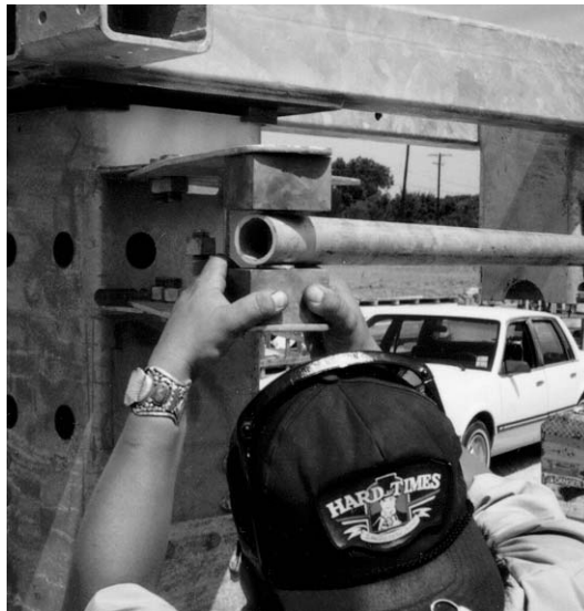
Figure 3-18: Azimuth Strut Assembly - Final Assembly
