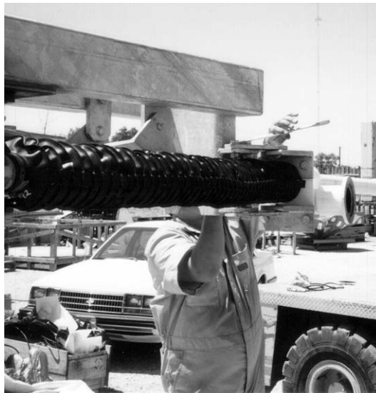
Figure 3-26: Protective Boot Attachment
