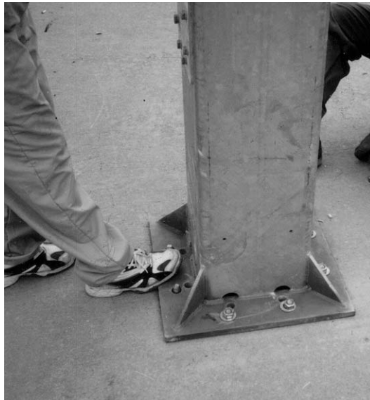
Figure 3-4b: Ground Mount Assembly Base Hardware
