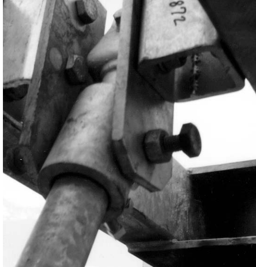
Figure 3-21a: Elevation Strut Bracket
