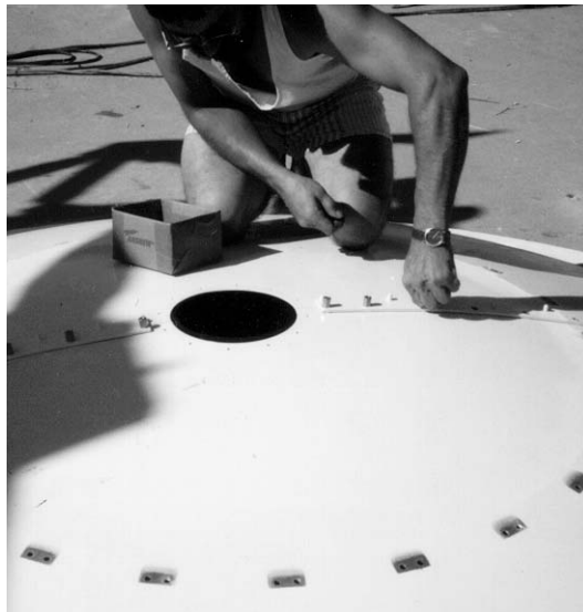
Figure 3-32: Seam Bolt Insertions
