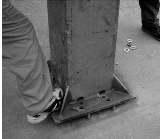
Figure 3-7: Mount Alignment/Adjustment
