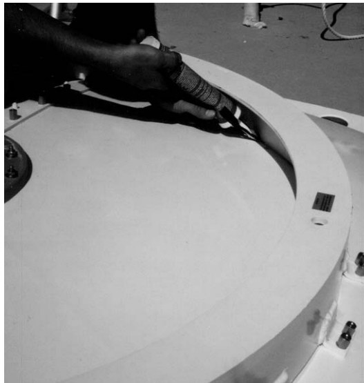
Figure 3-36: Mounting Ring Sealant (Equipment Enclosure Versions Only)
