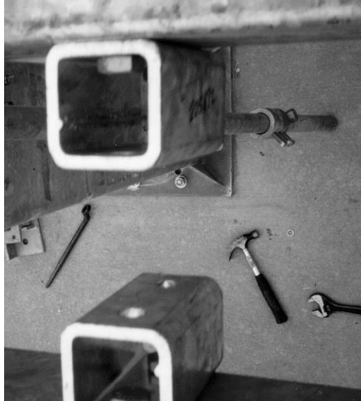
Figure 3-19: Elevation Strut Pick Up Assembly (Top View)
