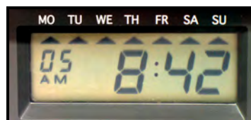
Figure 6-8. Failed Time Synchronization Display.
