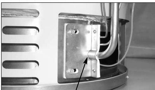
Radiused Channel for Feedline
