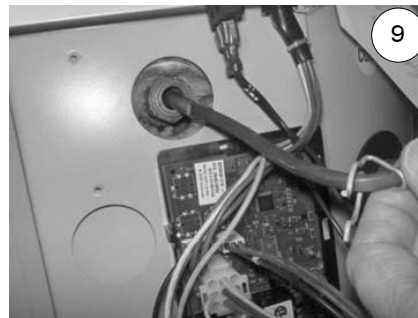
9 Removing lower sensor from well. Held in place by a clip fastened to well shoulder.
