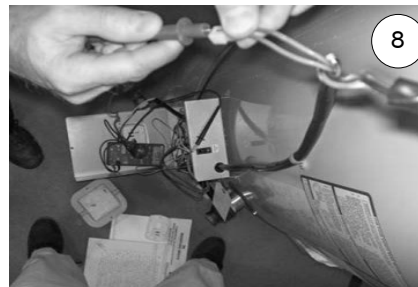
8 Checking continuity of upper sensor wire harness.
