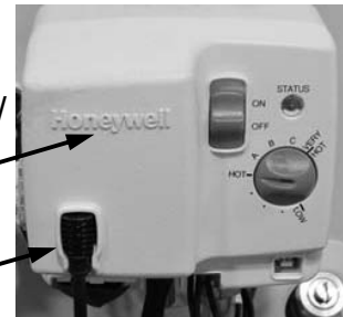
Spark igniter/flame sensor wire
