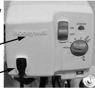
Spark igniter/flame sensor wire
