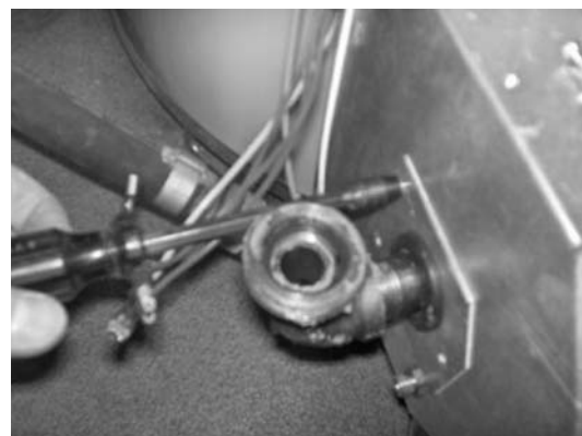
Step 6: Remove pipe flange plate from Burner Box
