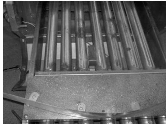
Step 14: Slide out burner assembly
