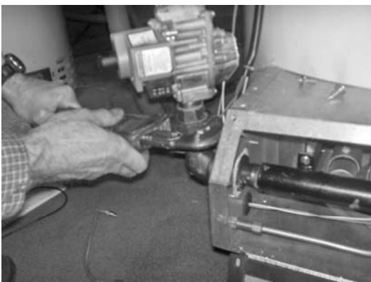
Step 5: Disconnect and Remove Gas Valve
