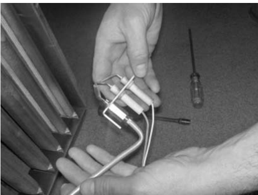
Step 17: Pilot removal for servicing.
