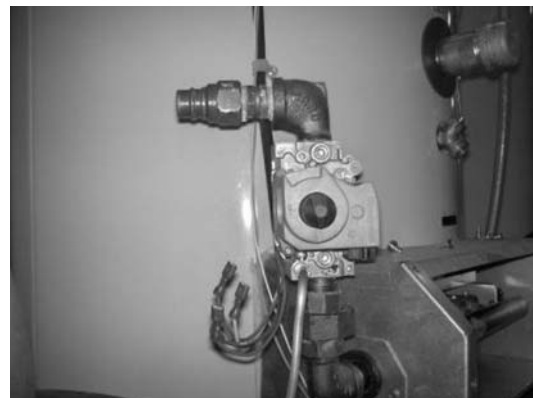
Step 4: Disconnect gas valve wires and pilot tube
