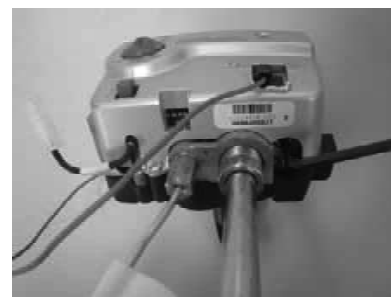
Gas Control shown in the "OFF" position
