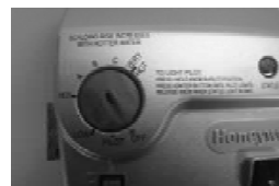
Gas Control shown in the "OFF" position
