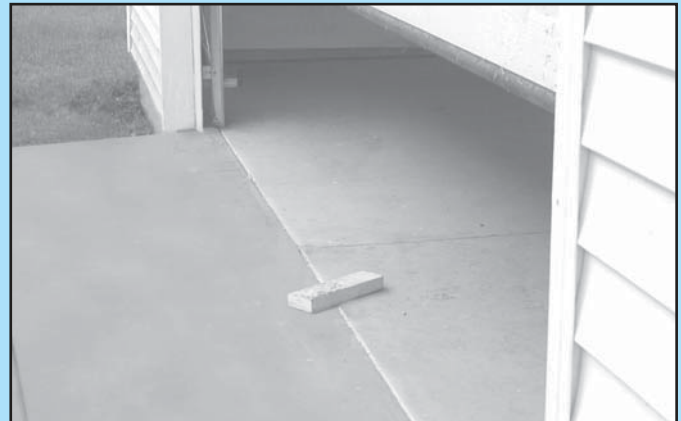
FIG. 6-6 2 x 4 under center of door opening.
