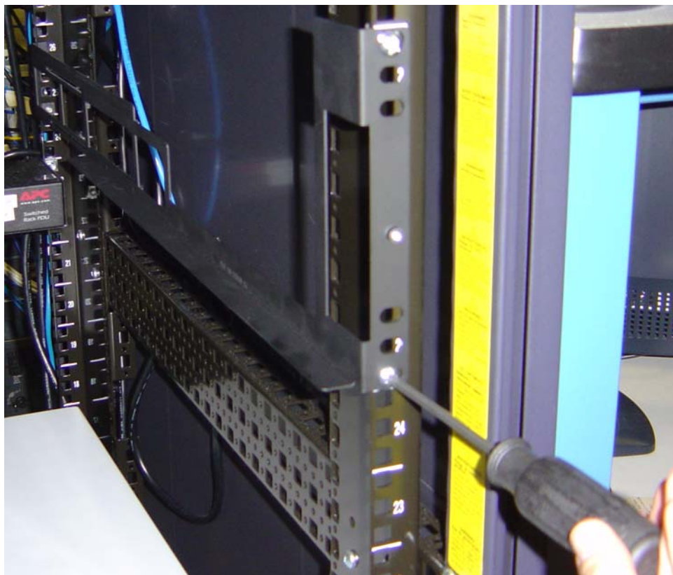
Figure 3-4: Attaching Rails from the Front
