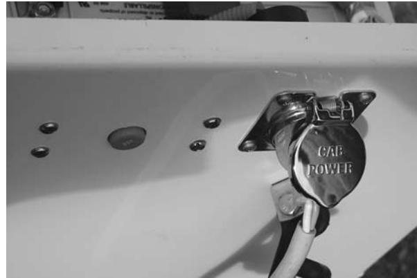
Figure 8 – Shorepower connection installed
