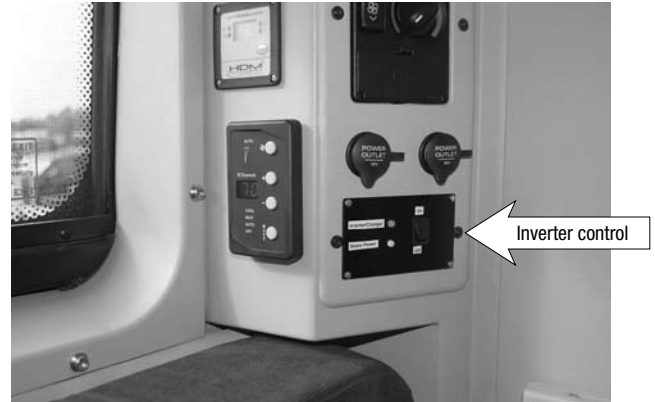
Figure 5 – Inverter control installed
