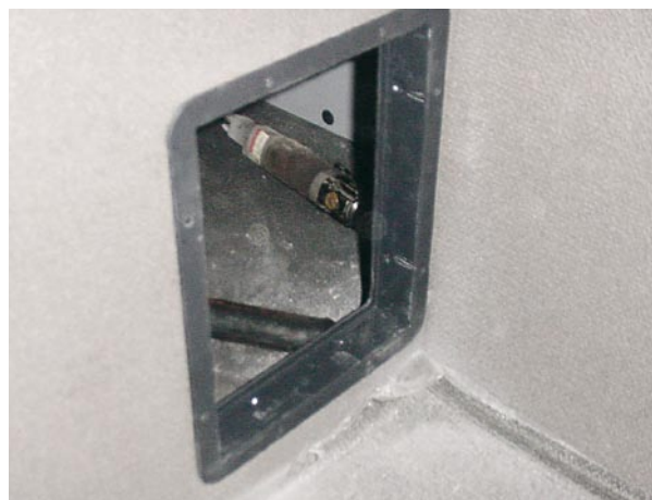
Figure 10 - Return air grill flange installed
