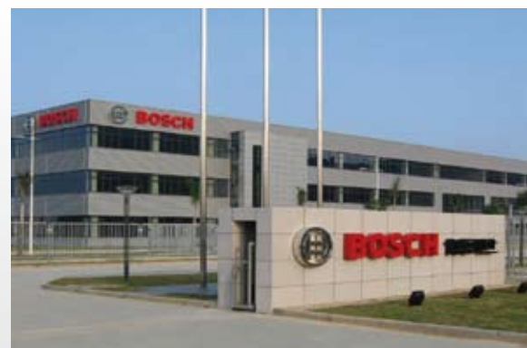
Manufacturing in Zhuhai, China
