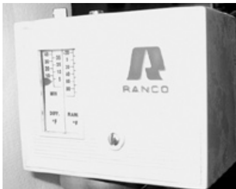
Thermostat located behind the On/Off switch panel.
