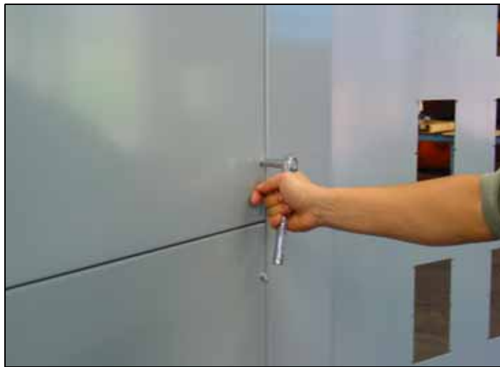
Figure 39. Removing the Bolts.
