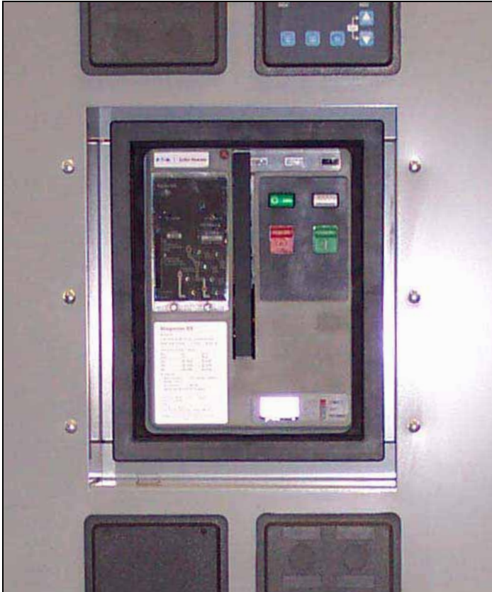
Figure 12. Insulated Case Switching Device.
