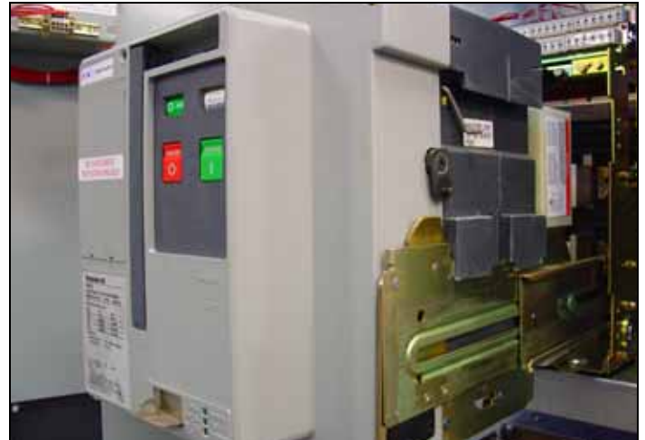
Figure 9. Drawout Switching Device Fully Extended from the Magnum Transfer Switch.
