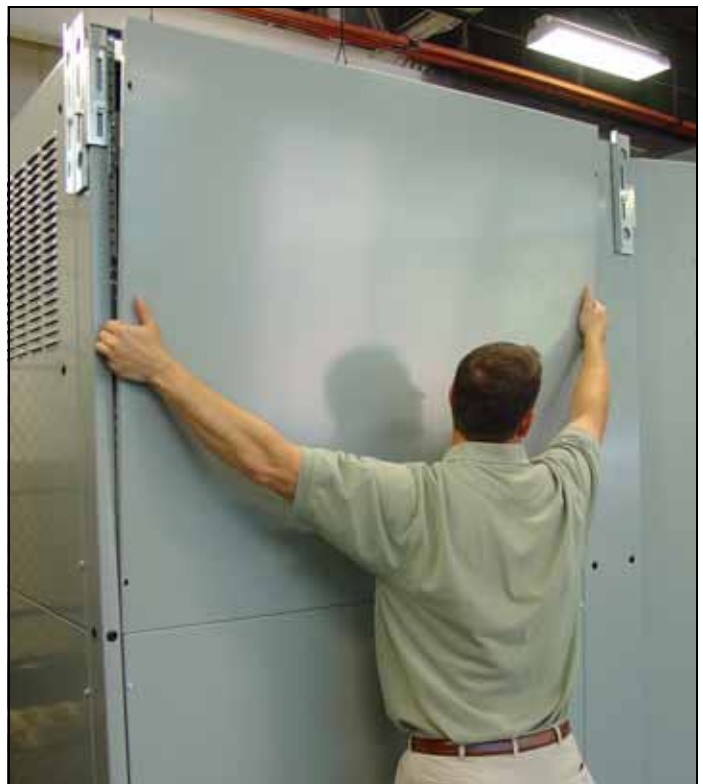
Figure 41. Lifting the Cover Free.
