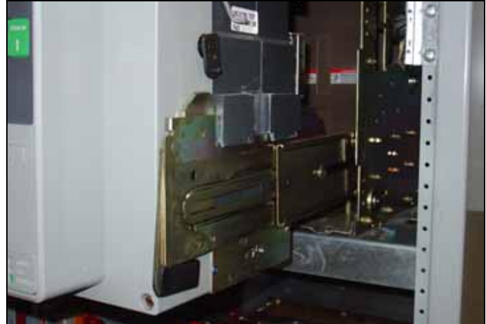
Figure 28. Switching Device in the REMOVE Position.
