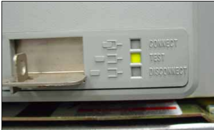
Figure 30. Switching Device in the TEST Position.
