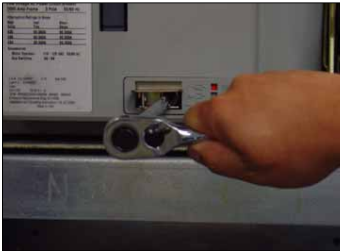
Figure 33. Levering and Position Indication.
