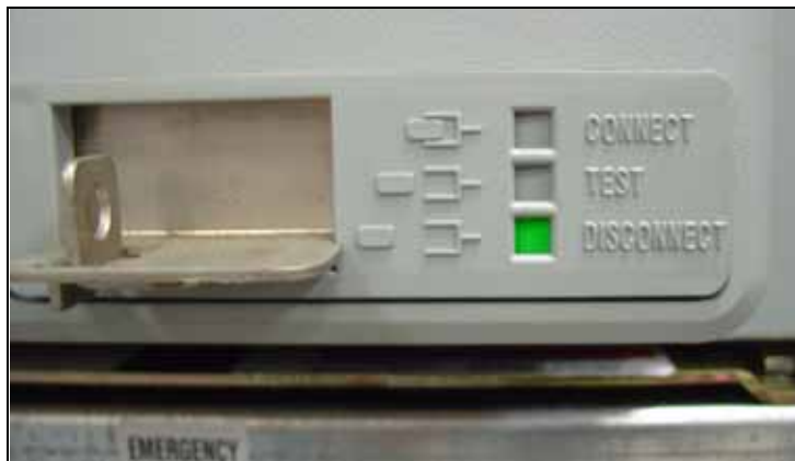
Figure 31. Switching Device in the DISCONNECT Position.
