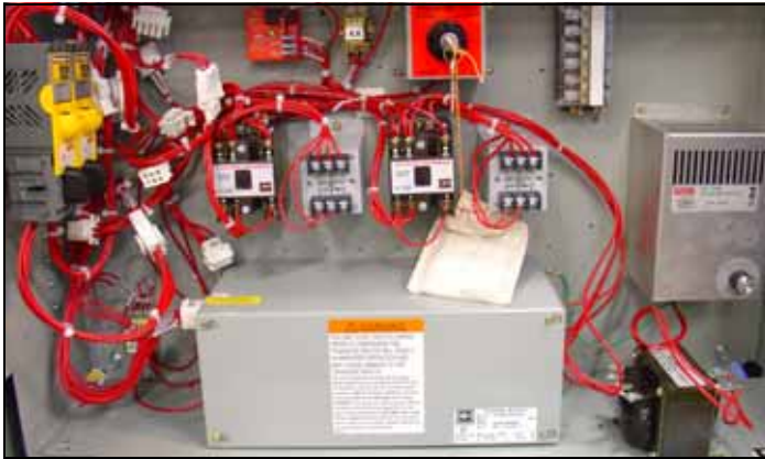
Figure 15. Voltage Selection Panel
