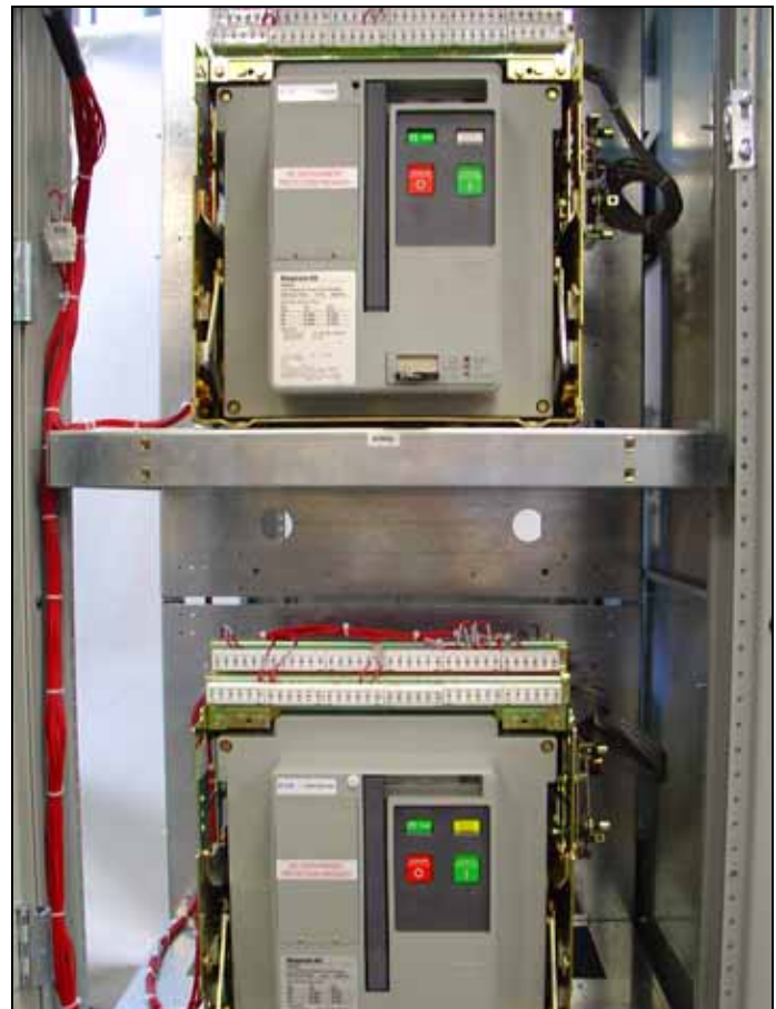
Figure 11. Typical Power Panel (Open Transition Shown).
