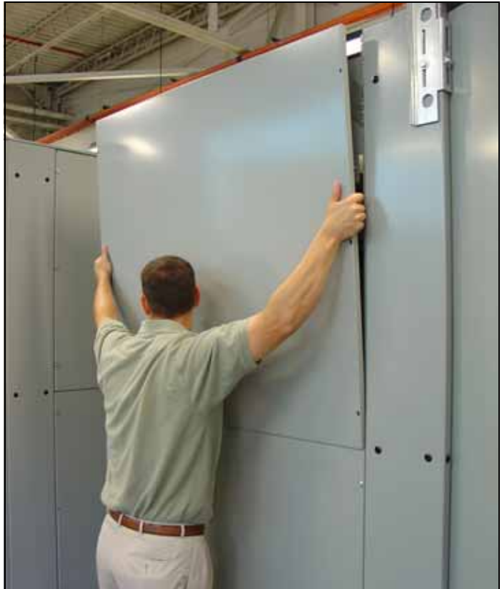
Figure 40. Tilting the Cover Away from the Frame.
