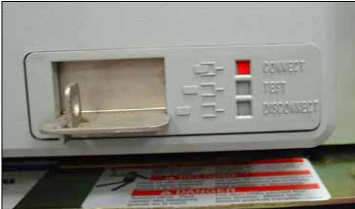
Figure 29. Switching Device in the CONNECT Position.
