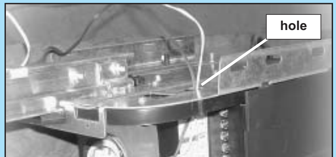
FIG. 1-12 Run wire to power head.
