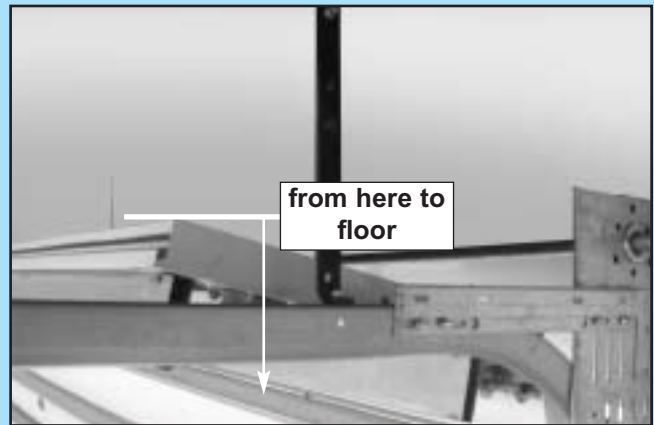
FIG. 2-1 Finding highest point of travel (sectional).
