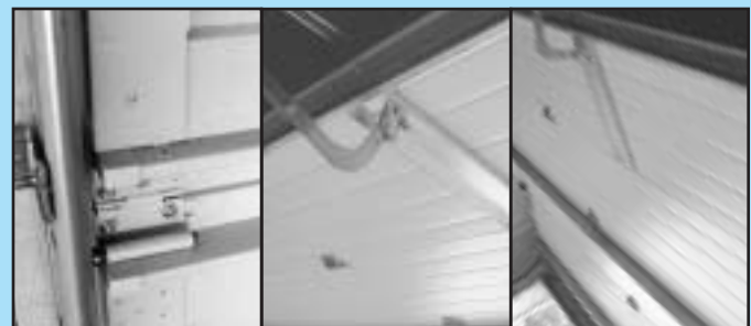
FIG. 2-6 Examples of door bracing.
